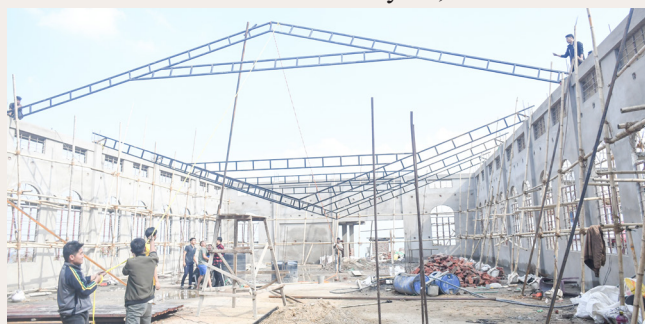
Students Helping in the Roof Construction of the New CTC Auditorium Hall
