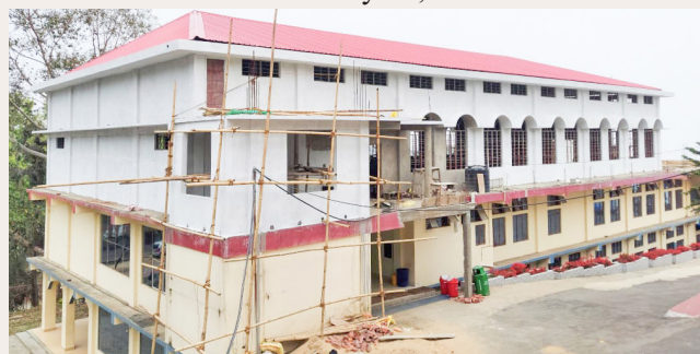
On going Construction of the New CTC Auditorium Hall
